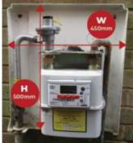
Back of Gas Box attached to wall (on which the Overbox will be attached to)
